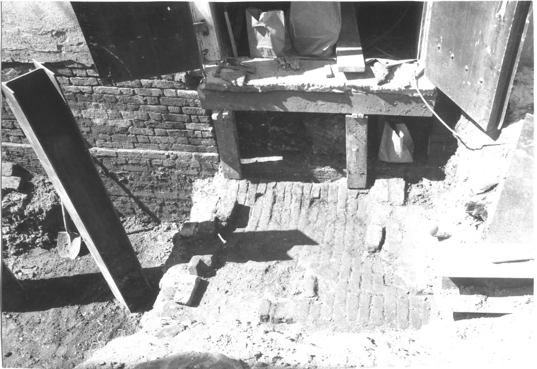
Figure 24. The original paving in front of the central cellar door on the east side of the Exchange Building.
